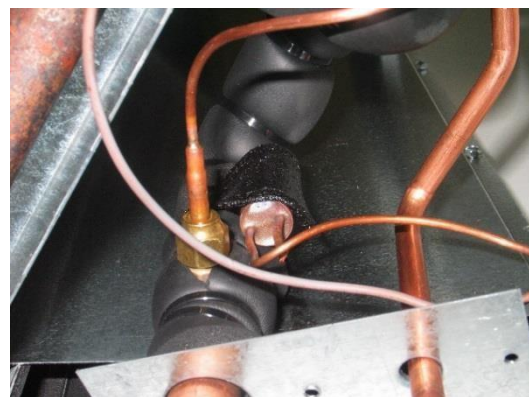
Figure 30. Bulb Secure Clamp and Cork Tape
