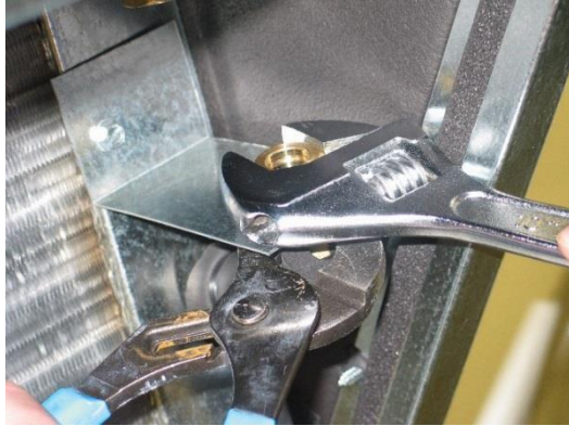
Figure 23. Remove Nut
