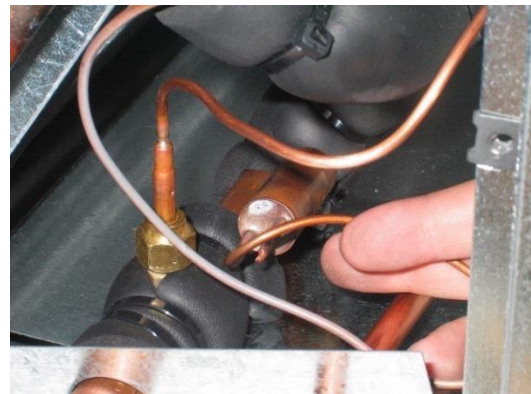
Figure 29. Thermal Measuring Bulb Placed on Copper Tube.
