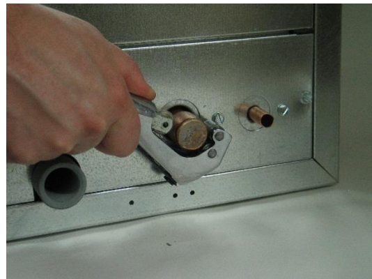
Figure 22. Cut end of connection as shown.
